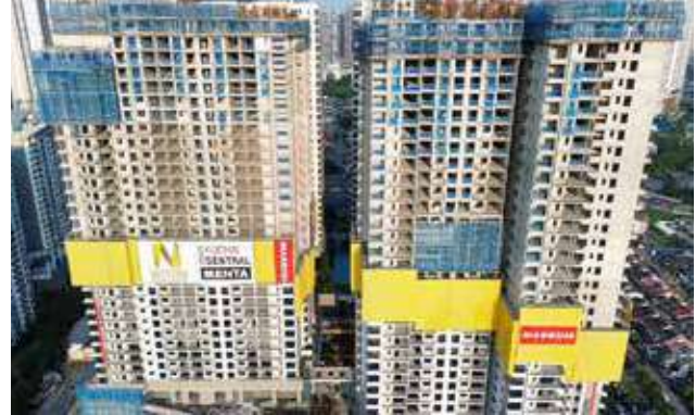
Kuchai Sentral Residence (Phase 2)
